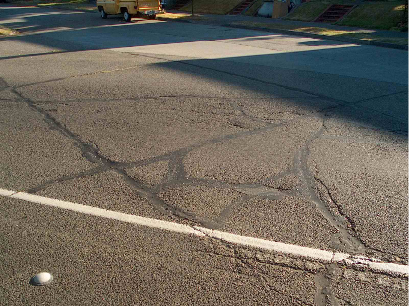
Asphalt Pavement Crack Repair
